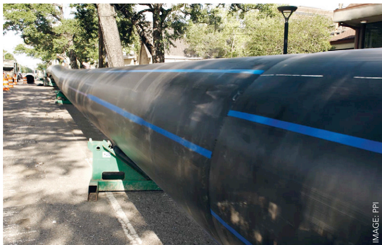
Above: A New Orleans project to replace water transmission mains used 4,400ft of 48in HDPE pipe from Agru
